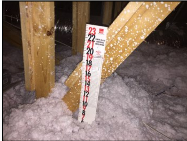
Attic insulation depth within recommended threshold.
